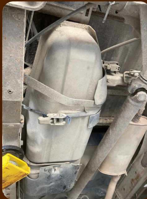
Missouri safety inspection found the fuel tank was strapped to the vehicle using a ratchet strap.
