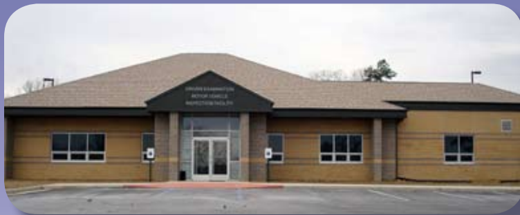
This building is part of a new CDL super site at the Troop I Headquarters in Rolla, MO.
