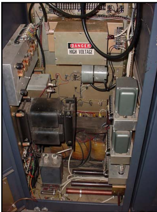
This picture is an example of outdated radio equipment still in service today in Missouri.
