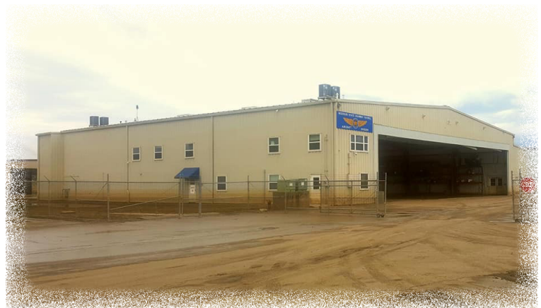
The flood damaged Patrol hangar is pictured on June 19, 2019.
