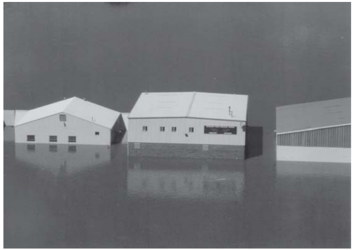
The Patrol's new aircraft hangar withstands its first test during a flood in 1995.
