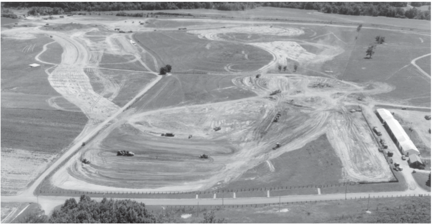
In September 1988, the Missouri National Guard completed work to bring the land up to grade for the Patrol's Defensive Driving Track.
