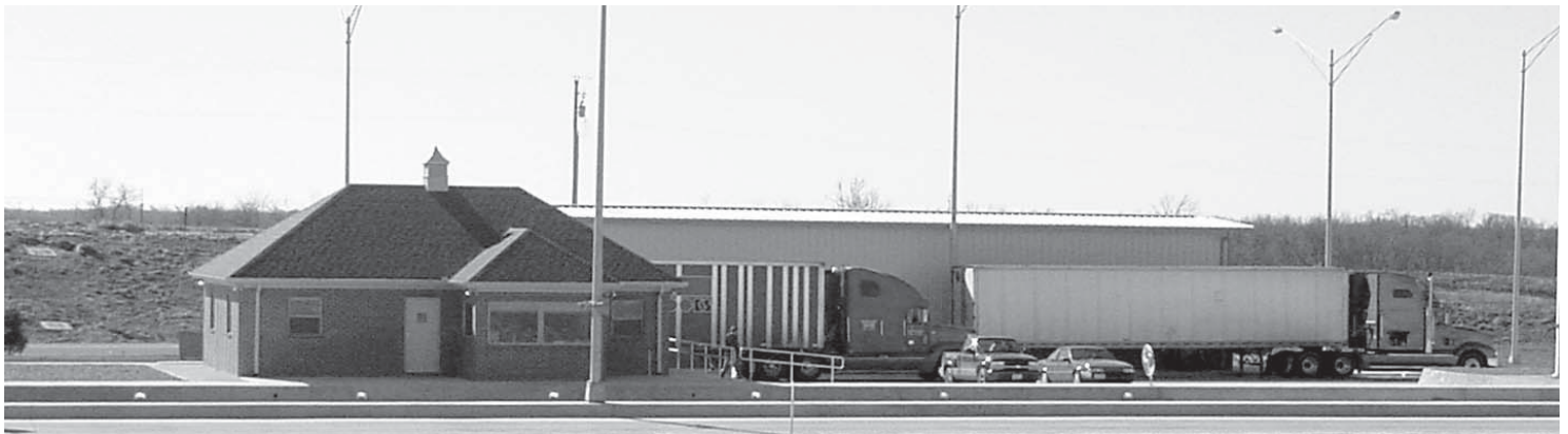
Pictured is the new A-3 scale house near Mayview, MO.
